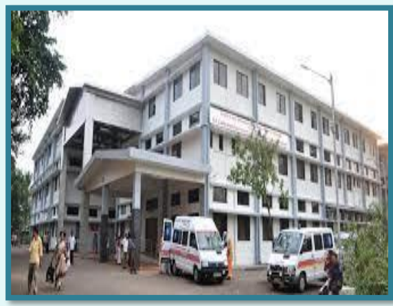
Bhaktshreshtha Kamalakar pant Laxman Walawalkar Hospital, Dervan Ratnagiri
